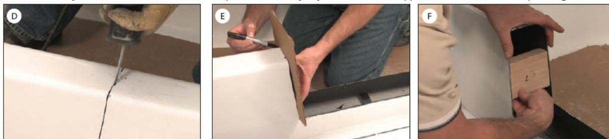
Step 14: Hold a 2 x 4 halfway up the opening and trace lines on both sides of the opening onto the 2 x 4 marking the width. Mark the 2 x 4 so you know if it is the left or right side. Do the same for the opposite side, then cut the wood according to the markings.
