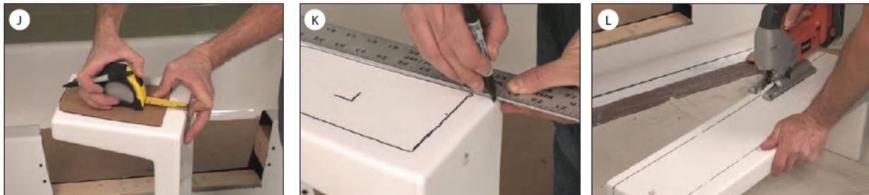
Step 28: After proper fit is accomplished, take off the insert. Add a liberal amount of adhesive to the wood blocks on each side and on top of the stack of wood resting on the floor. Do not apply adhesive directly to the insert at this time. Push the insert into place.
